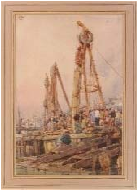
Pile Driver at Rouen
